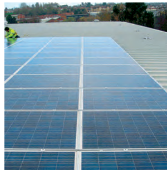
Solar panel installation, Reading
