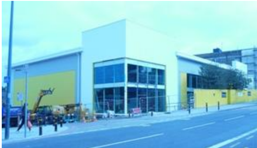
Store under construction
