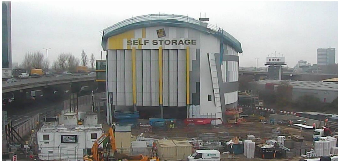
Store under construction
