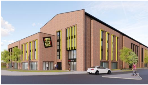
Hove, under construction
