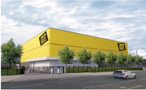
Harrow, under construction
