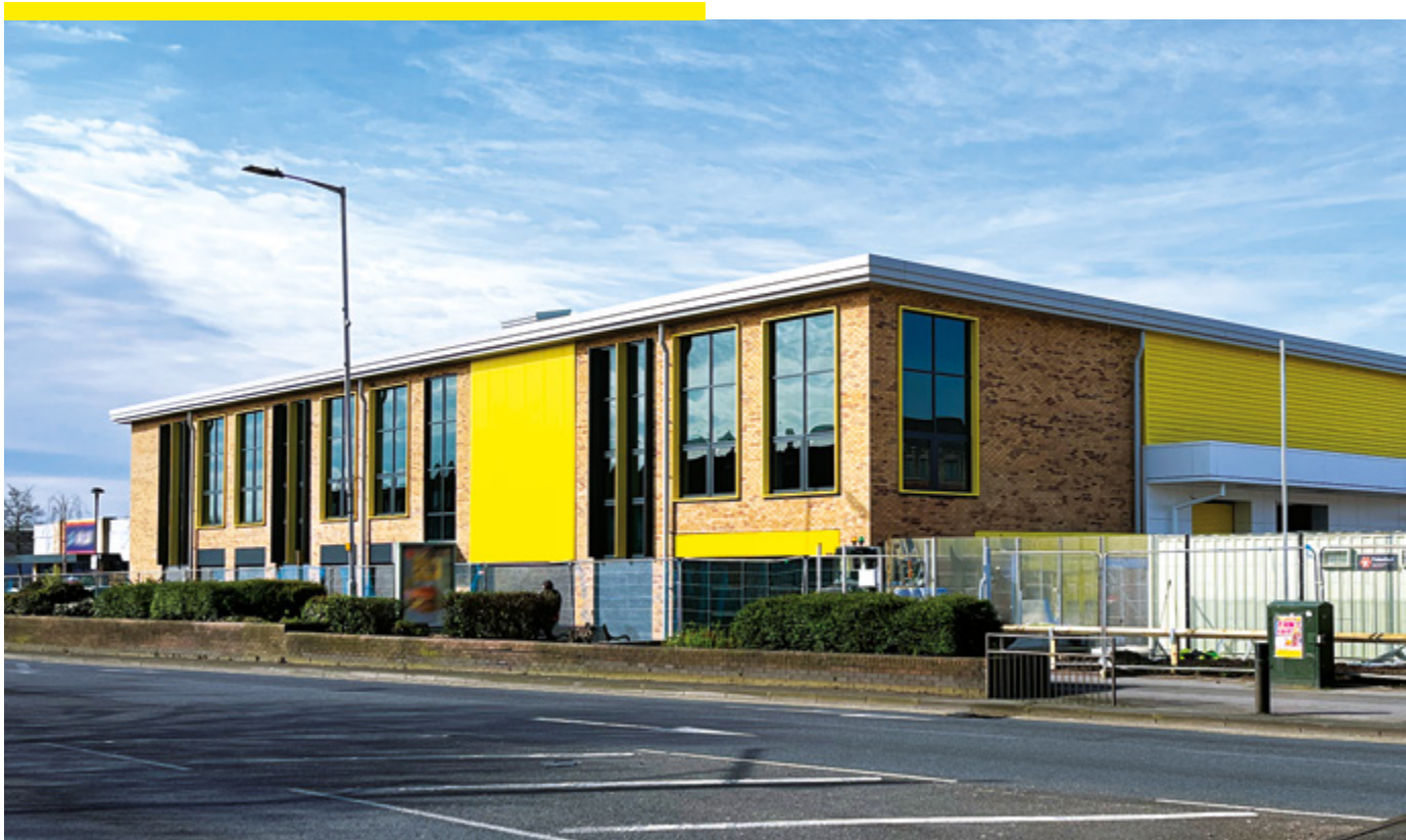
Big Yellow Slough Farnham Road under construction – opening July 2024
